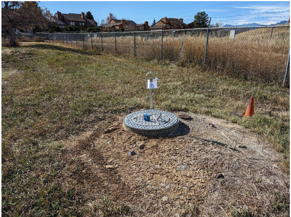
Photo 6. N. Water Treatment Plant
