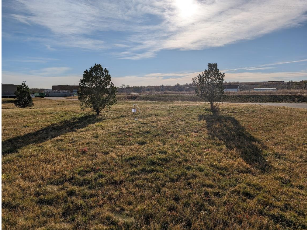
Photo 7. Wastewater Treatment Plant
