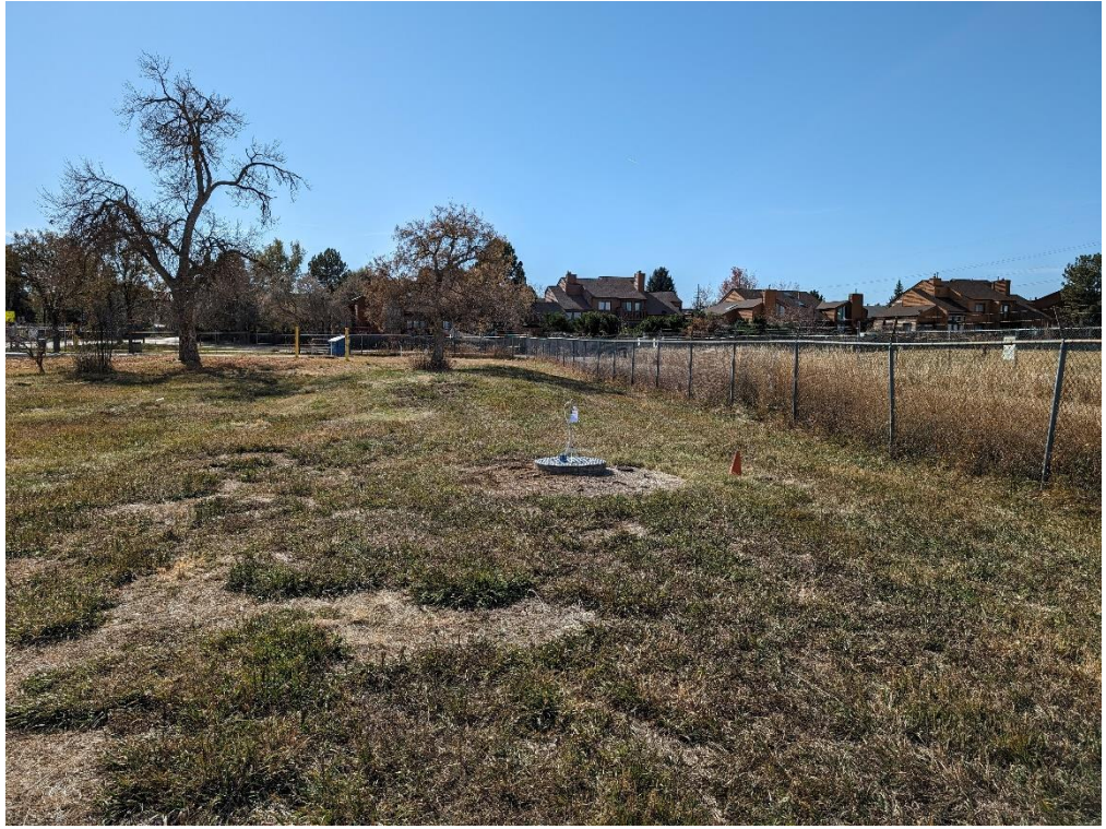
Photo 5. N. Water Treatment Plant
