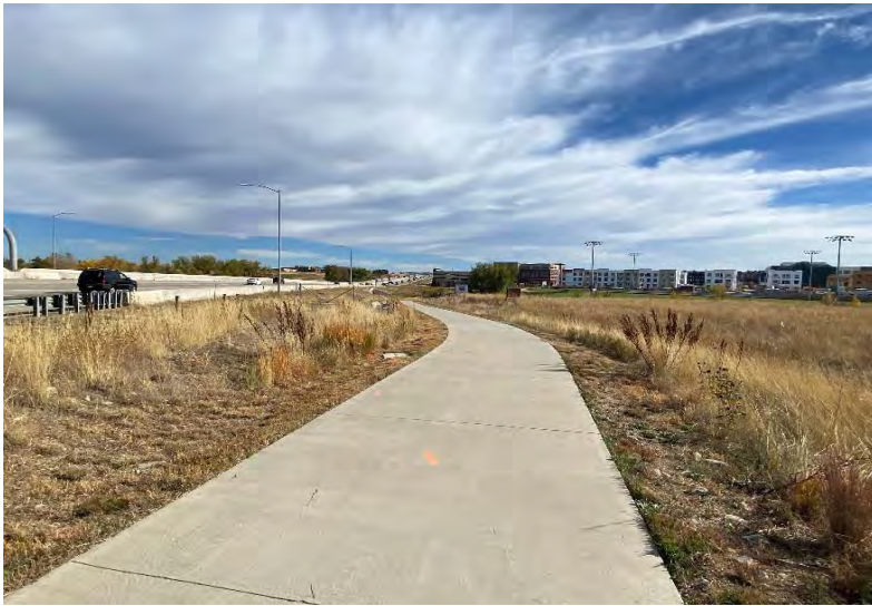
View along the eastern border of the subject site, shared with walking trail, followed by a drainage culvert and US Highway 36. View to the south.
