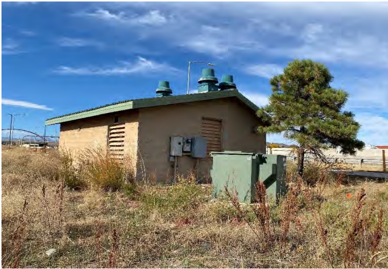
View of northerly adjoining utility building. View to the north.
