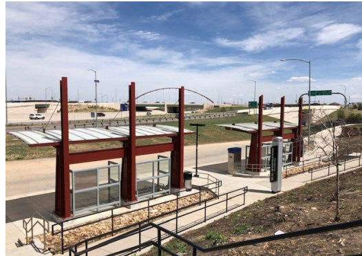
Existing: RTD Station
