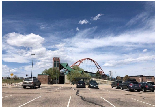
Existing: McCaslin Bridge
