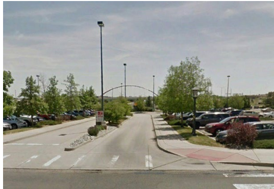
Existing: Center Drive
