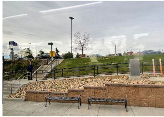
Existing: RTD Station
