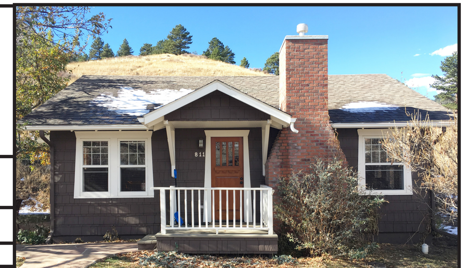
ASPHALT, PITCHED ROOF BRICK MATERIAL GABLED ROOF FORM ENTRY ELEMENT BRACKETS AT ROOF ENTRY ELEMENT MISSION STYLE DOOR AND EXTERIOR LIGHTS
