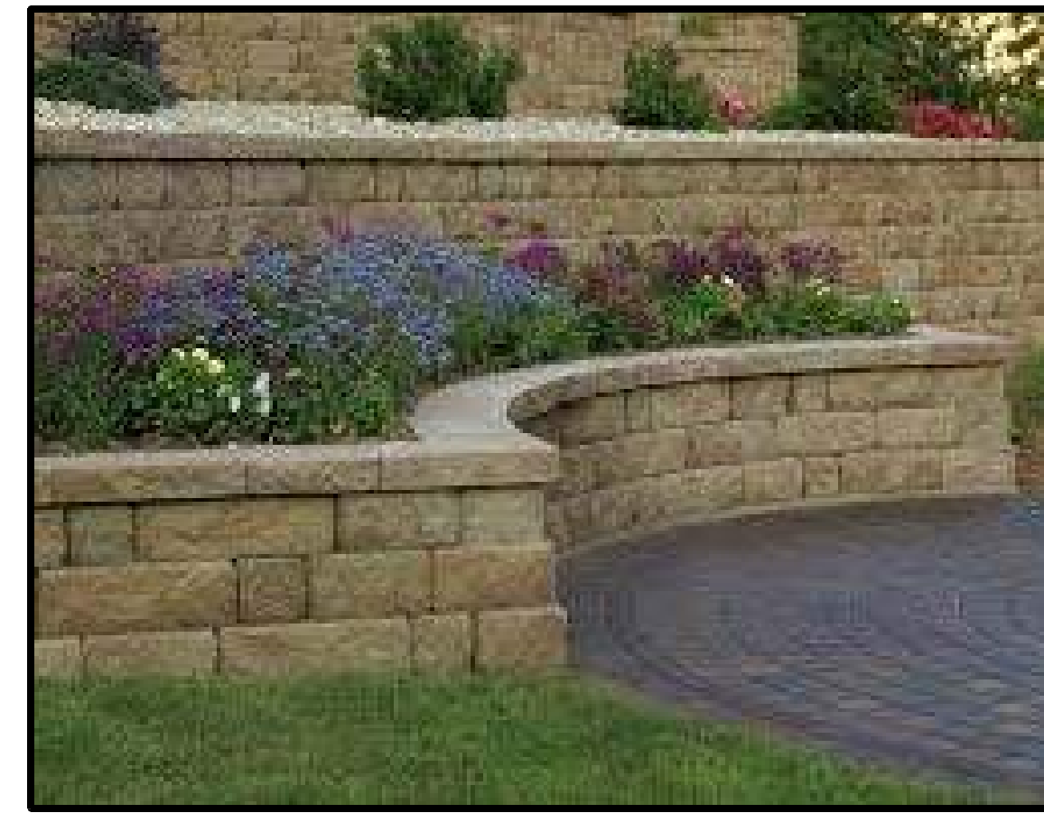
Masonry Block Retaining Wall Wall Height Varies - See Drainage Plan for Wall Height. Structural Design may vary at time of construction.
