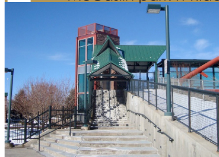
Pedestrian Bridge at McCaslin park-n-Ride
