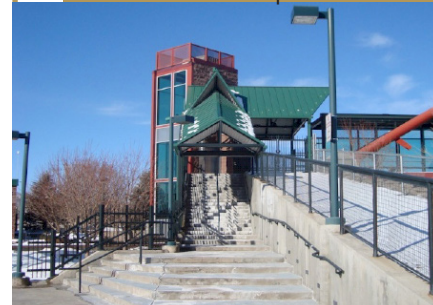
Pedestrian Bridge at McCaslin park-n-Ride
